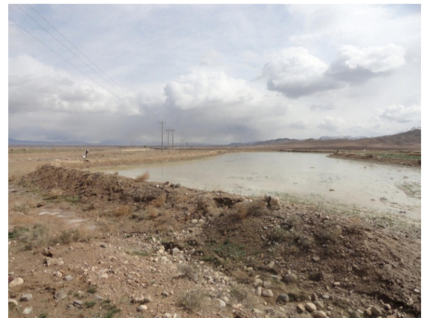
Fig. 4. The incoming water spreads behind levees so that the resulting backwater makes the soil moisture to increase to a sufficient level for sustaining compatible cultivation.
