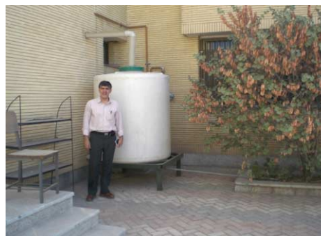
Figure 9 | Roofwater downpipe and collection tank (First author is standing next to the raintank).
